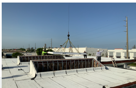
Oversized Skylight Installation
