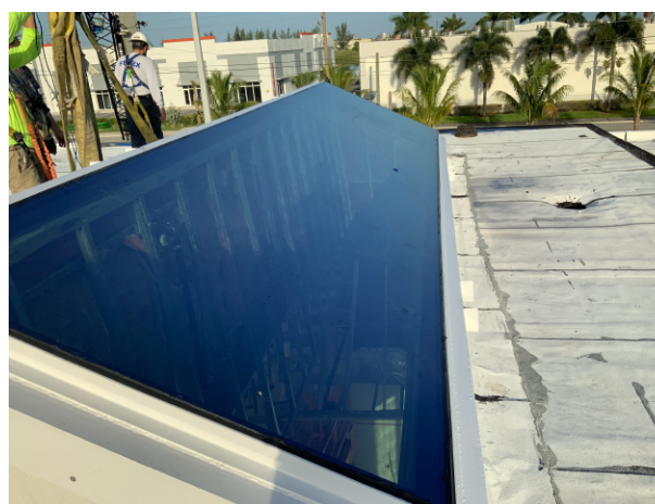
Installed 4'-10" W x 19'-3" Skylight
